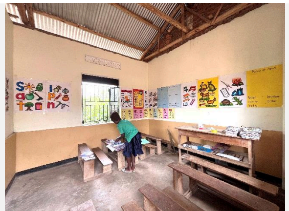
Figure 11 A photo of one of the class rooms after repair.
