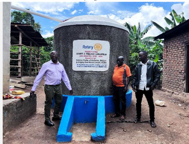
Figure 14 Some of the completed Tanks.
