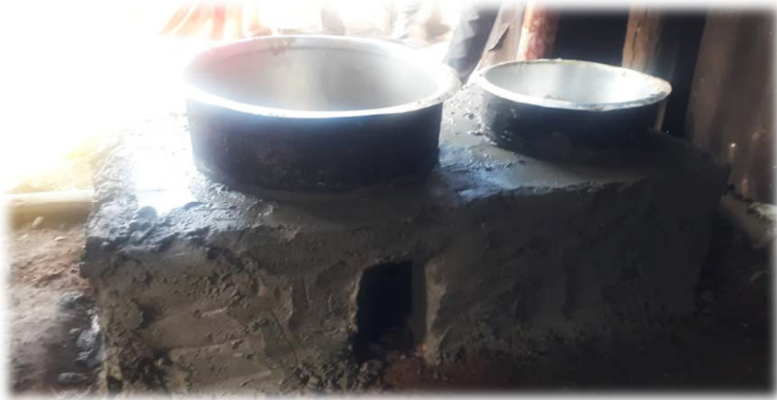
Figure 79 Fuel saving stoves under construction.
