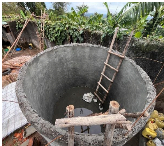
Figure 12 Some of the photos showing RWH tank construction progress.
