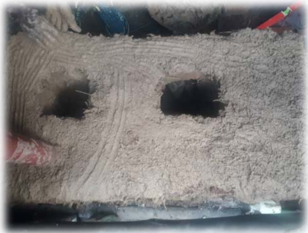
Figure 82 Some of the stoves under construction.
