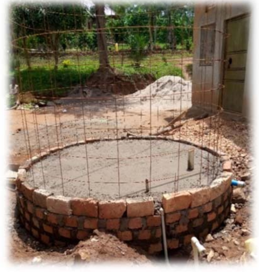
Figure 23 Setting of the Tank
