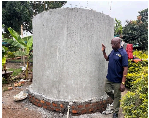
Figure 13 Rtn. Kyaluzi FX participating in the monitoring of tanks construction.
