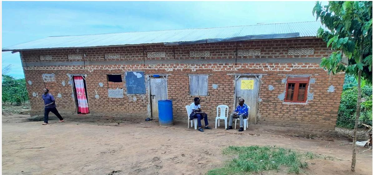
Figure 8 A photo of Harvest Primary school before repair.
