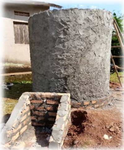
Figure 24 Shell wall Construction in progress.
