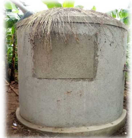
Figure 26 Tank under Curing
