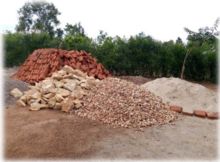
Figure 22 Part of the Materials used for construction.
