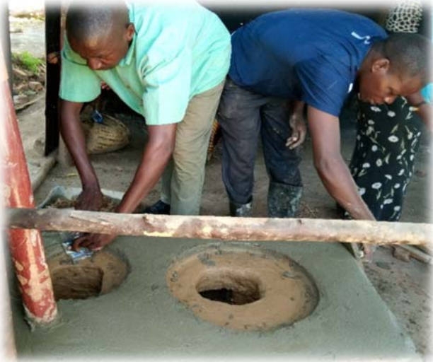
Figure 80 Stoves under Construction.
